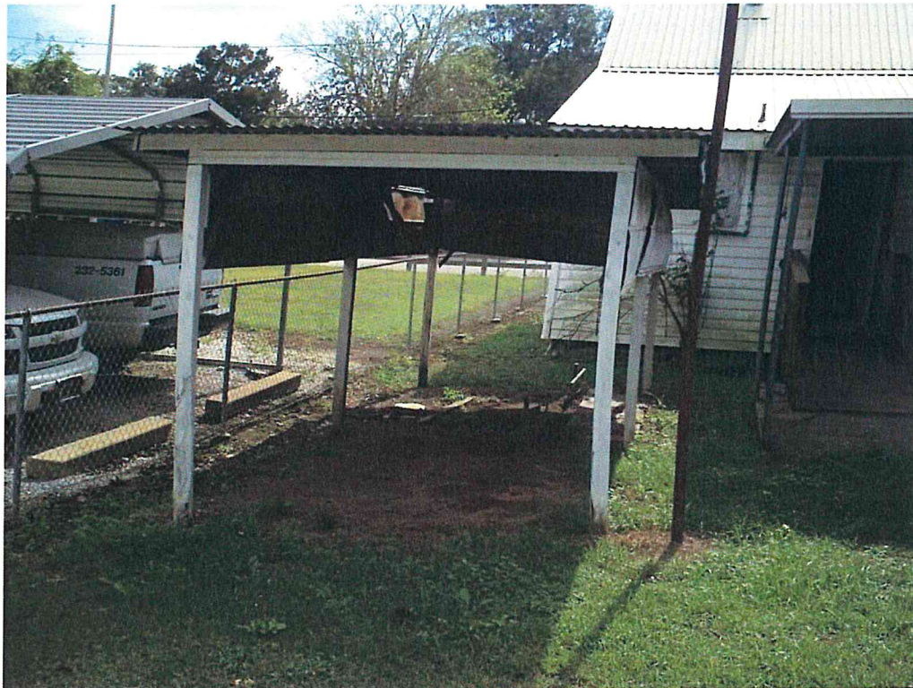
Photo 1 View of structure.
