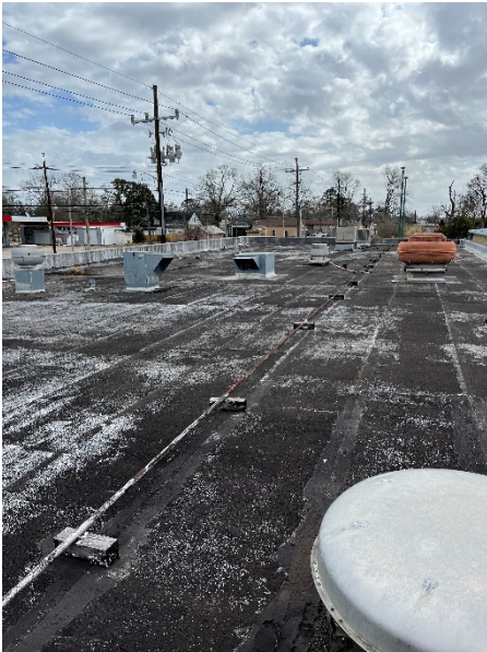
Photo of building roof where the parapet wall was sampled.
