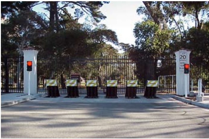
Figure 1: Use of Active and Passive Barriers
