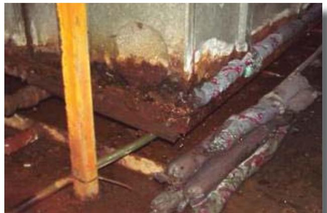
Damage on the Exchanger due to cooling water leak
