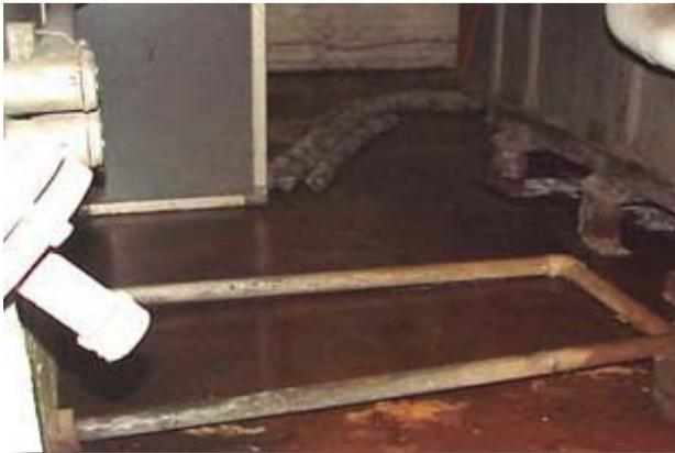
Flooding in the mechanical room from cooling water leak
