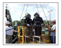
**TO#03:** Divers penetrated into valve pit and cleaned seal at Old River Lock. Utilizing crane and man basket, divers lowered 50' to reach water, then work in 25' water depth to clear isolation gate.
