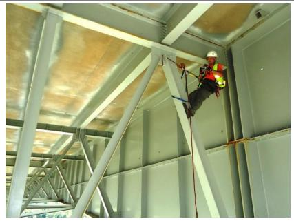
accurately measure significant section loss and other deterioration that affects member capacity. Drones/UAV's are also utilized to augment inspection capabilities.
