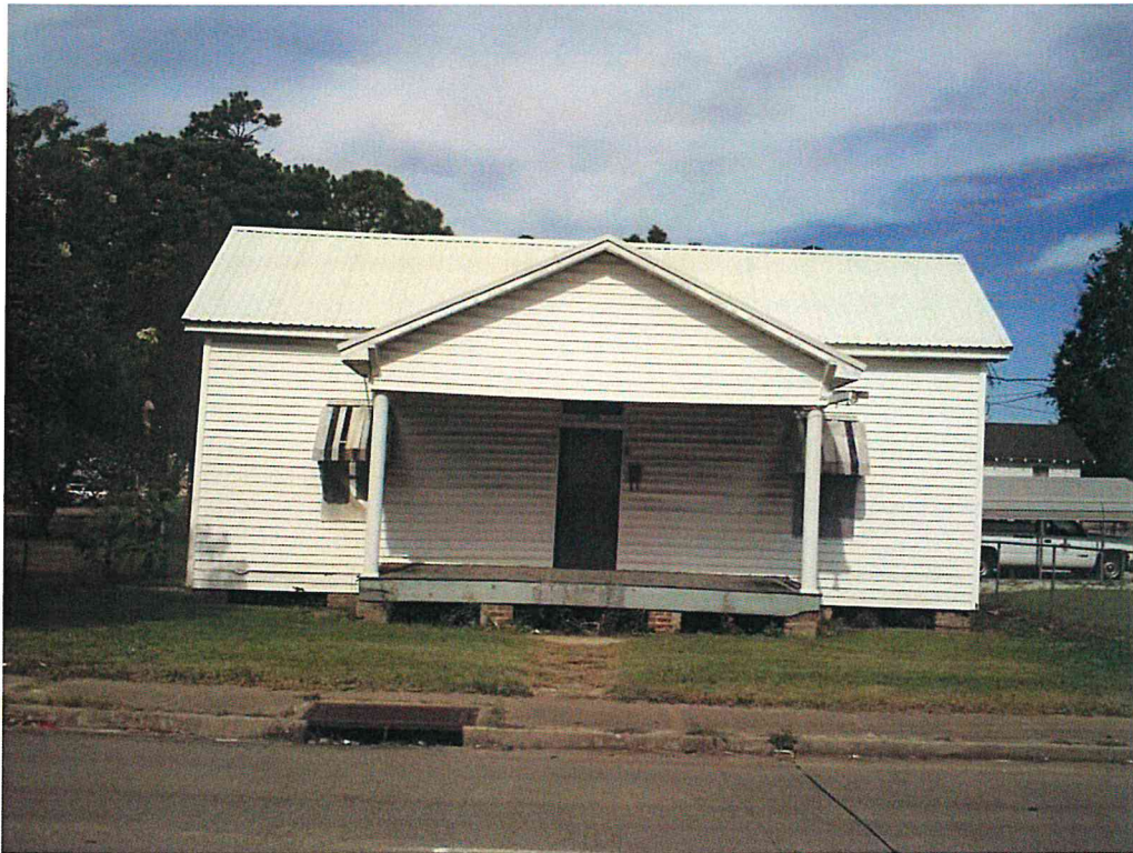
Photo 1 View of structure.
