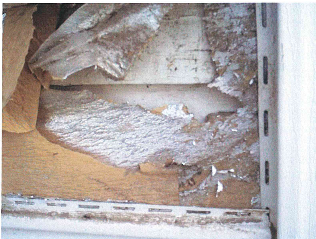
Photo 4 View of HA-3: Non-ACM paper between exterior vinyl siding and wood siding.
