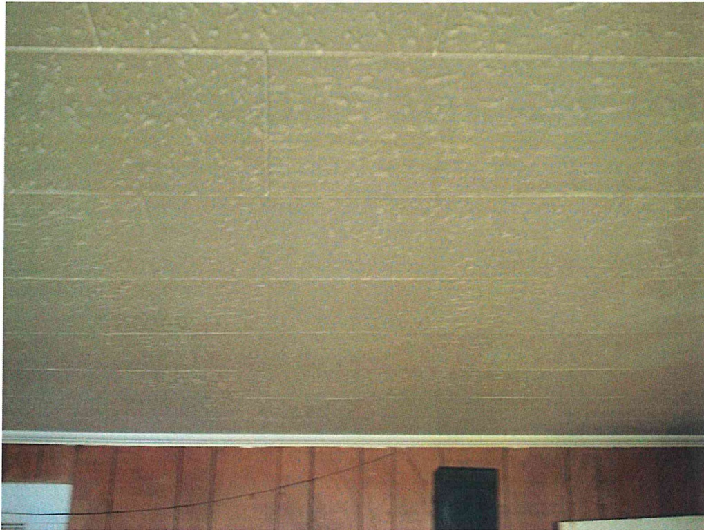
Photo 5 View of HA-5: Non-ACM interlocking textured ceiling tile.
