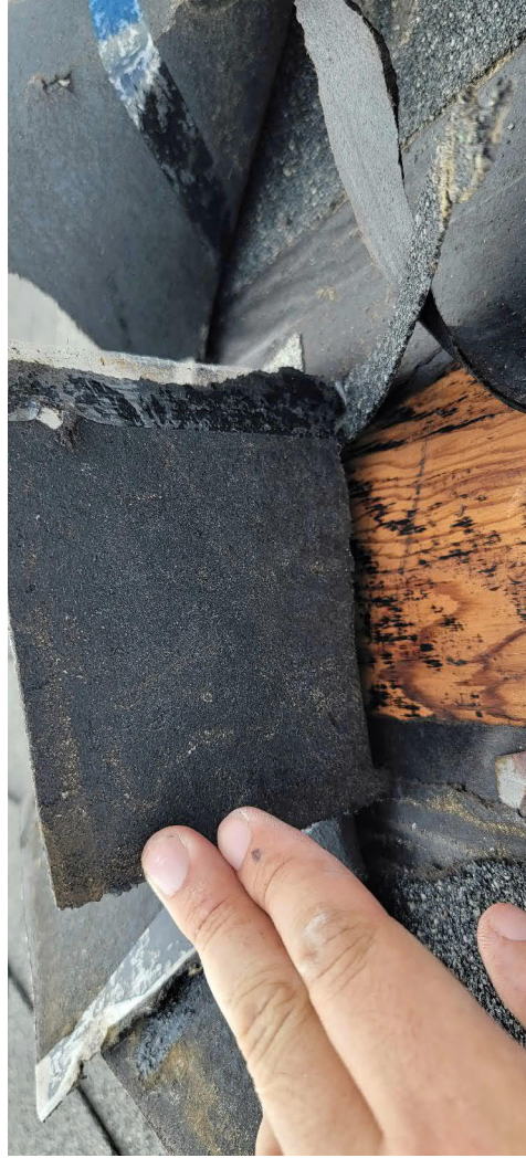
Photograph No. 9 HA-09: Black Roof Shingles with Black Tar Paper
